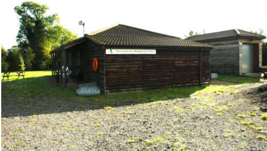
View of the Field Centre in 2006 with extension to the nearside and tractor store in the background.
